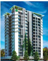
DD HIGHWAY GATE
